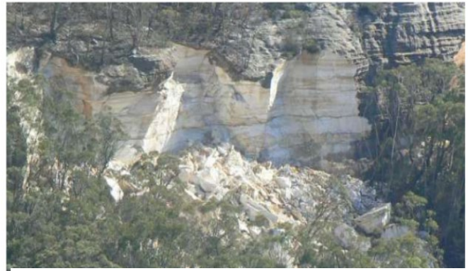
Maximum damage cliff fall, Baal Bone Colliery. Photo by D. Burgess, 2007.
